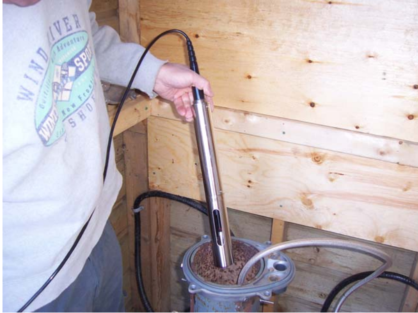
A Hydrolab sonde being lowered down a well.
