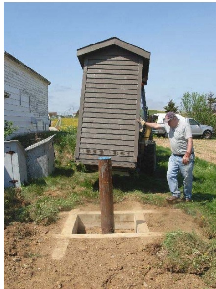
Observation well hut installation
