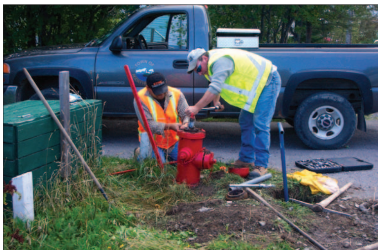
Operators maintain a fire hydrant in Rocky Harbour
